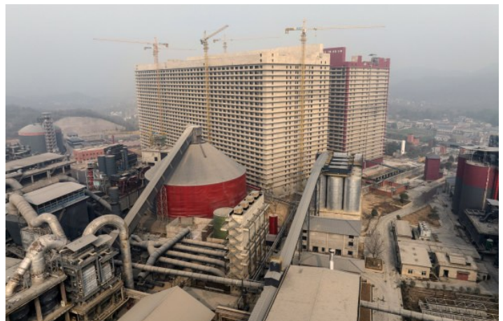
The 26-storey building on the outskirts of Ezhou, China is being hailed as the world's biggest free-standing pig farm with a second identical hog high-rise opening soon.C
