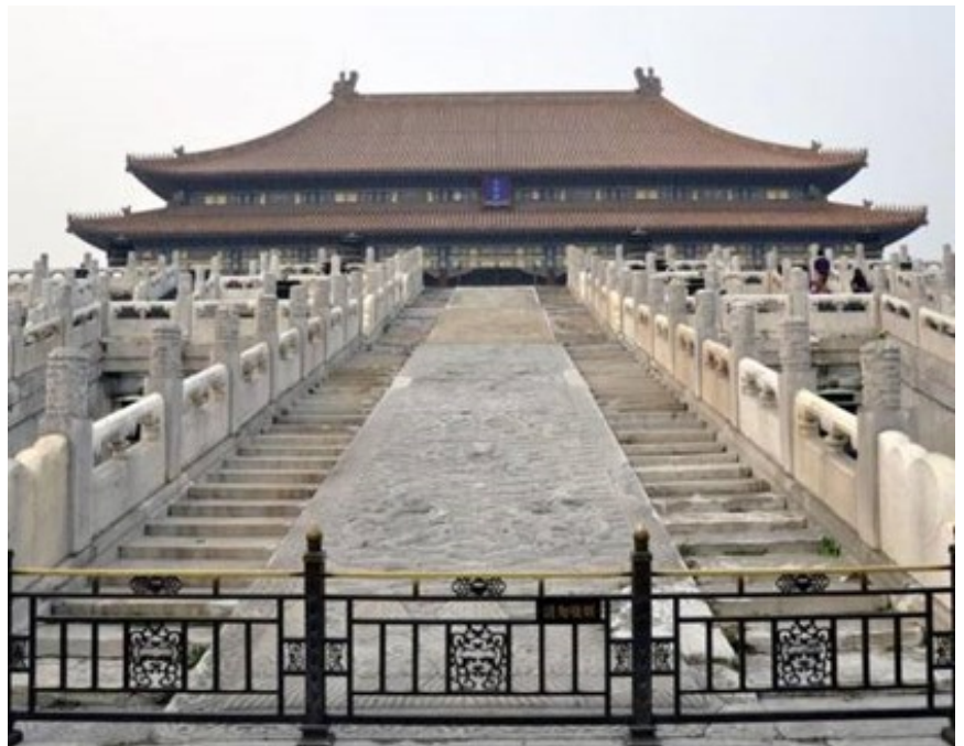
Hall of Supreme Harmony, Forbidden City Records show ancient Chinese workers pulled the 300-ton centre stone in this famous staircase over man-made roads of ice. (Credit: Image courtesy of Chui Hu)
