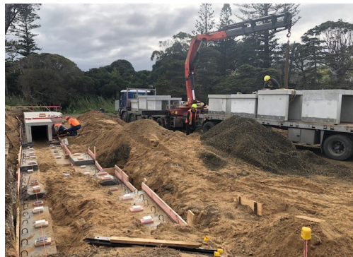
Laying of foundations to support steps
