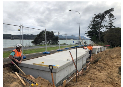
First of concrete steps in position
