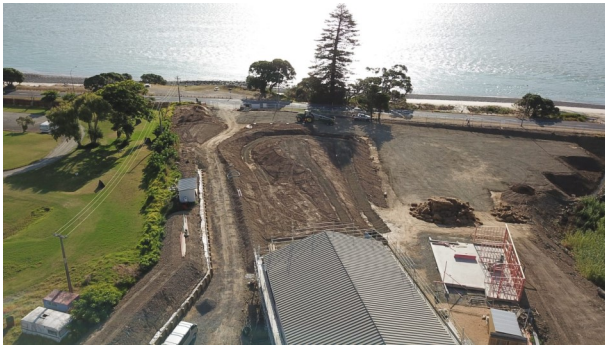
Aerial view of site
