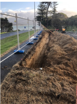
Beginning of foundations
